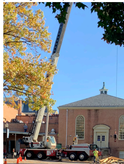
Crane placing HVAC equipment on the roof before starting construction
